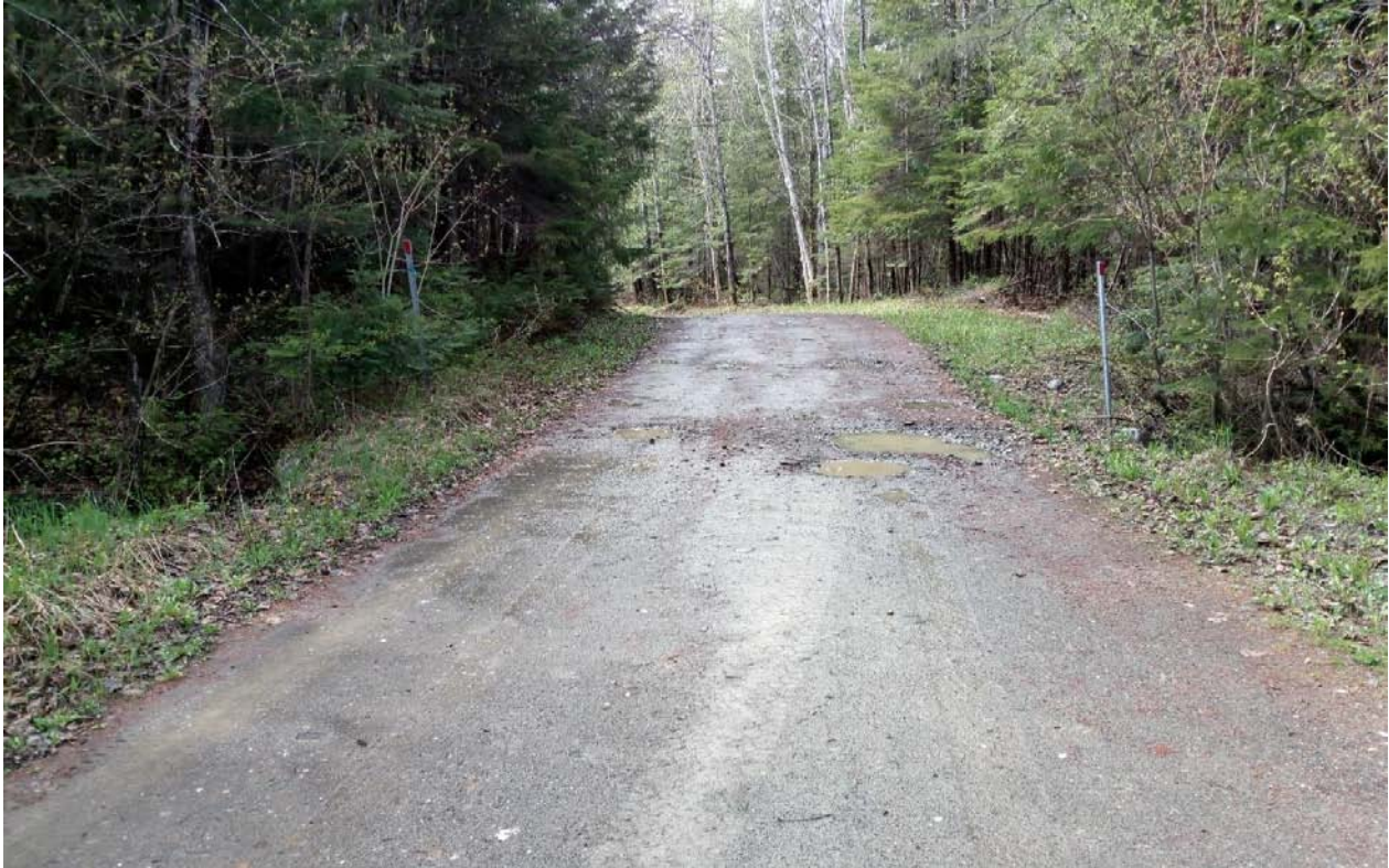
Photo 23 Remblais insuffisants
