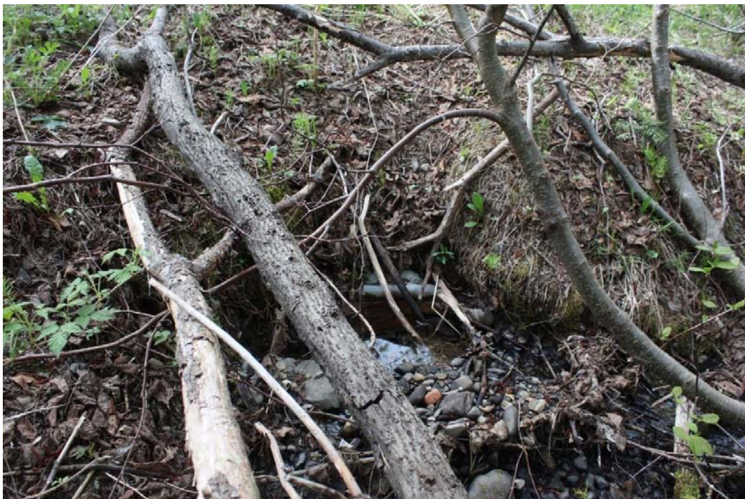
Photo 41 Ponceau obstrué, 35-DR2
