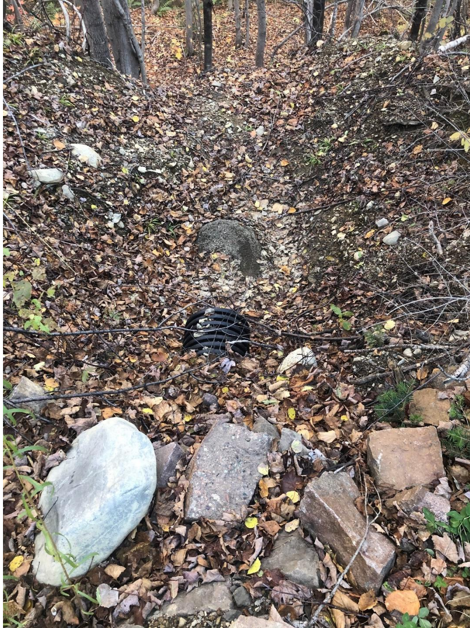
Photo 44 Ponceau obstrué, R-DR26
