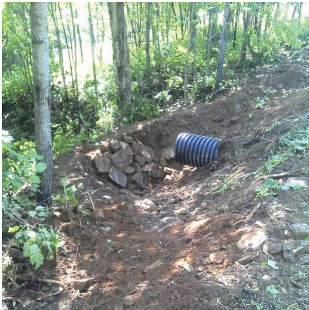
Figure 32. C70-DR3 – Ponceau de drainage installé
