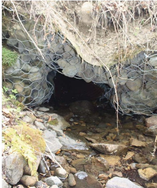
Figure 1. Remblai aval instable
