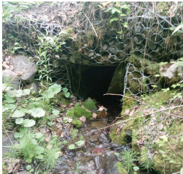
Figure 2. Remblai amont instable
