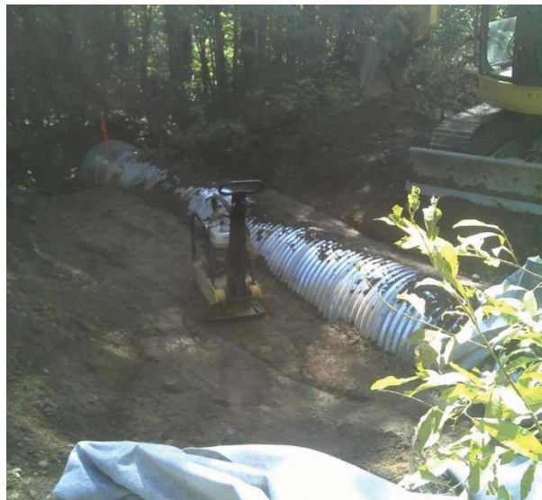
Figure 10. Installation du ponceau
