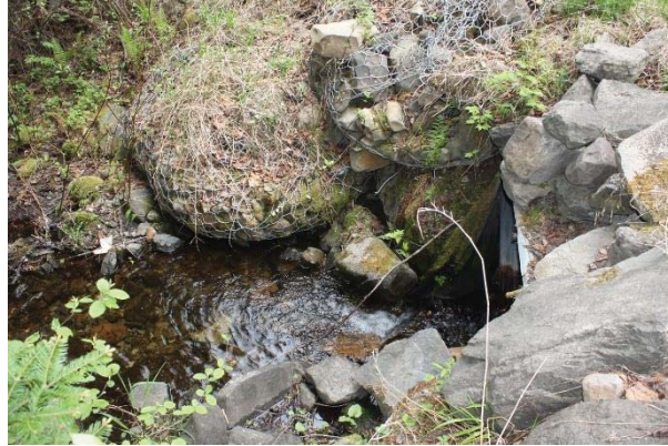
Figure 9. Caissons de roches instables
