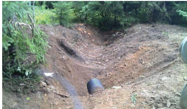
Figure 22. Bassin de sédimentation, C70-DR7.5-IMP
